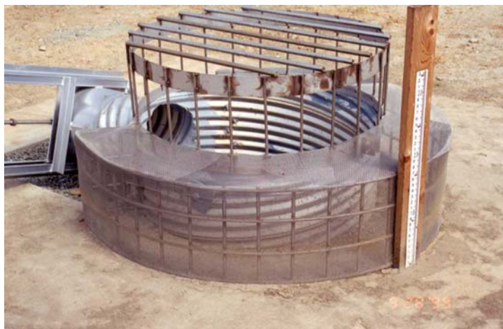
Figure 1 Example of Extended Detention Outlet Structure
