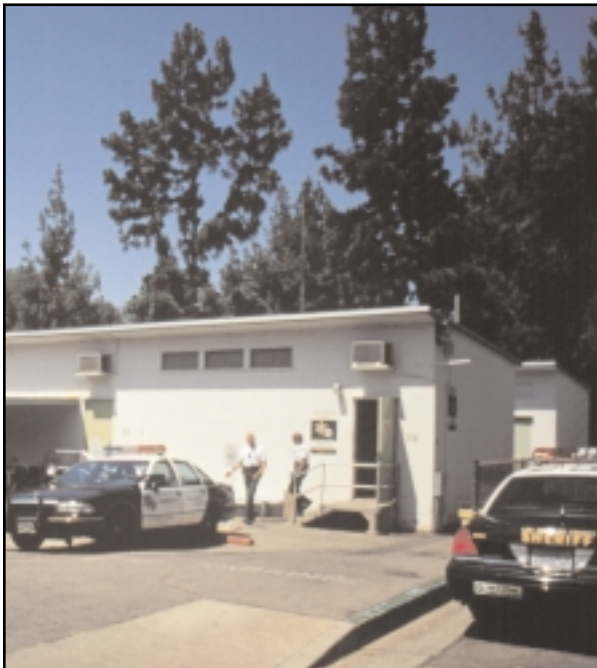
Existing Campus Sheriff Station in bungalow.
