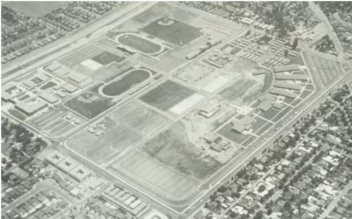
Figure A 0-6. Aerial view of the campus around 1960.
