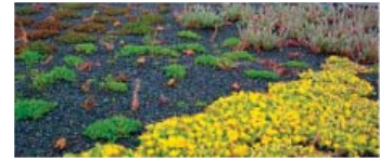
Sedum Planted Green Roof
