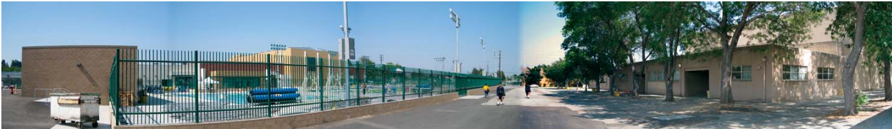
Aquatics Complex and South Gym
