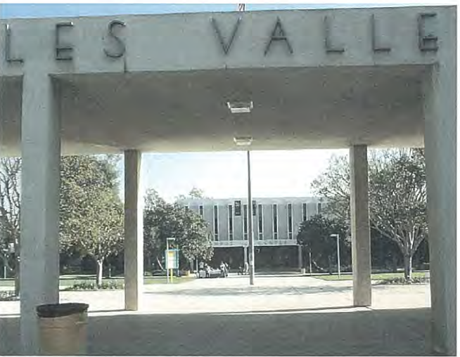
View into the Campus Core
