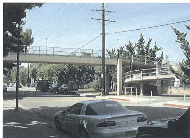
Closed Pedestrian Bridge on Ethel Avenue
