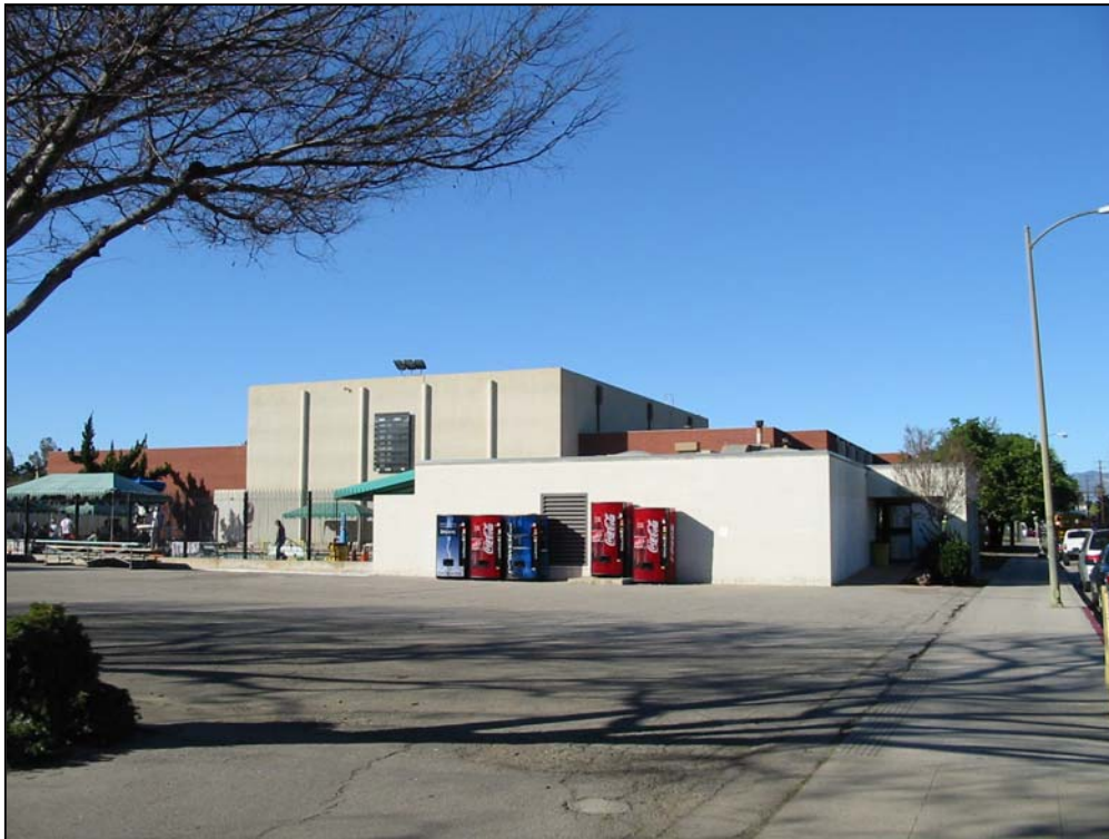
Figure 3-16: Paved Area Adjoining North Gym, Looking North
