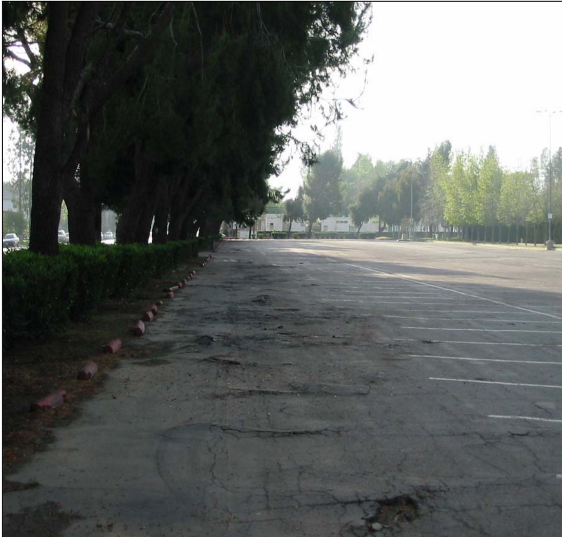
Figure 3-11: Parking Lot G, Looking East (Landscape Unit B)
