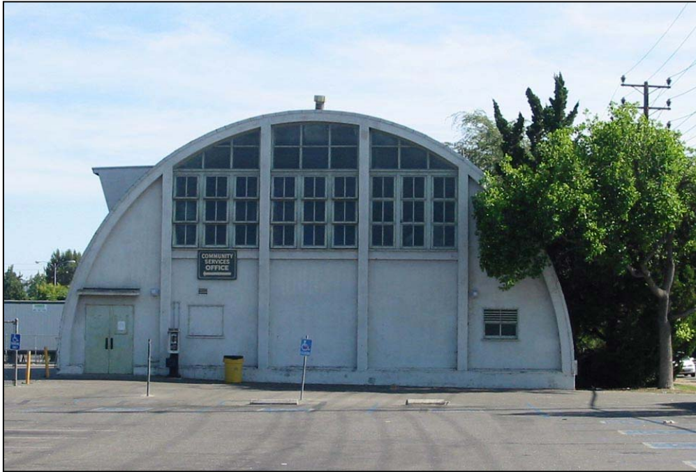
Figure 3-15: Field House (Original 1952 Gymnasium)
