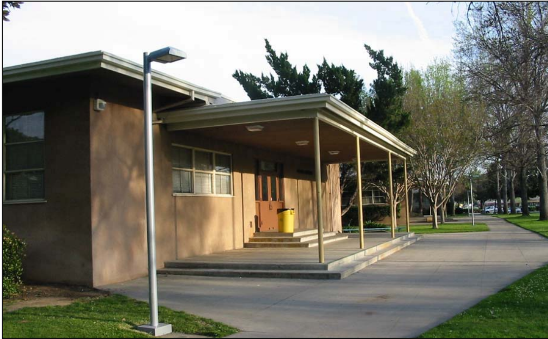
Figure 3-30: West Façade of Chemistry Building, Looking South
