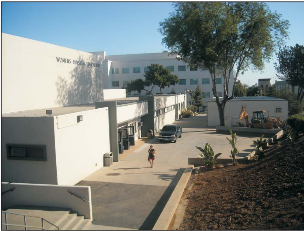
Women's Gym. Light beige and green concrete exterior, symmetrical rectangular forms with a flat roof and minimal window openings.
