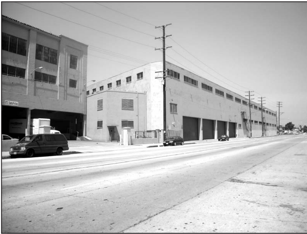
View of the east-facing facade of Buildings 3 and 4 located on the eastern project site from Santa Fe Boulevard.
