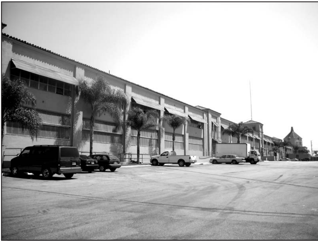
View of the south-facing facade of Building 1 located on the eastern project site from Firestone Boulevard.
