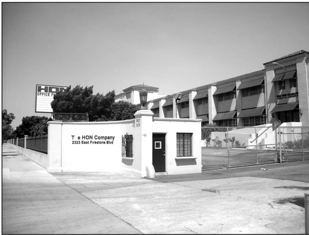
View of the south-facing facade of Buildings 1 and 2 located on the western project site from Firestone Boulevard.
