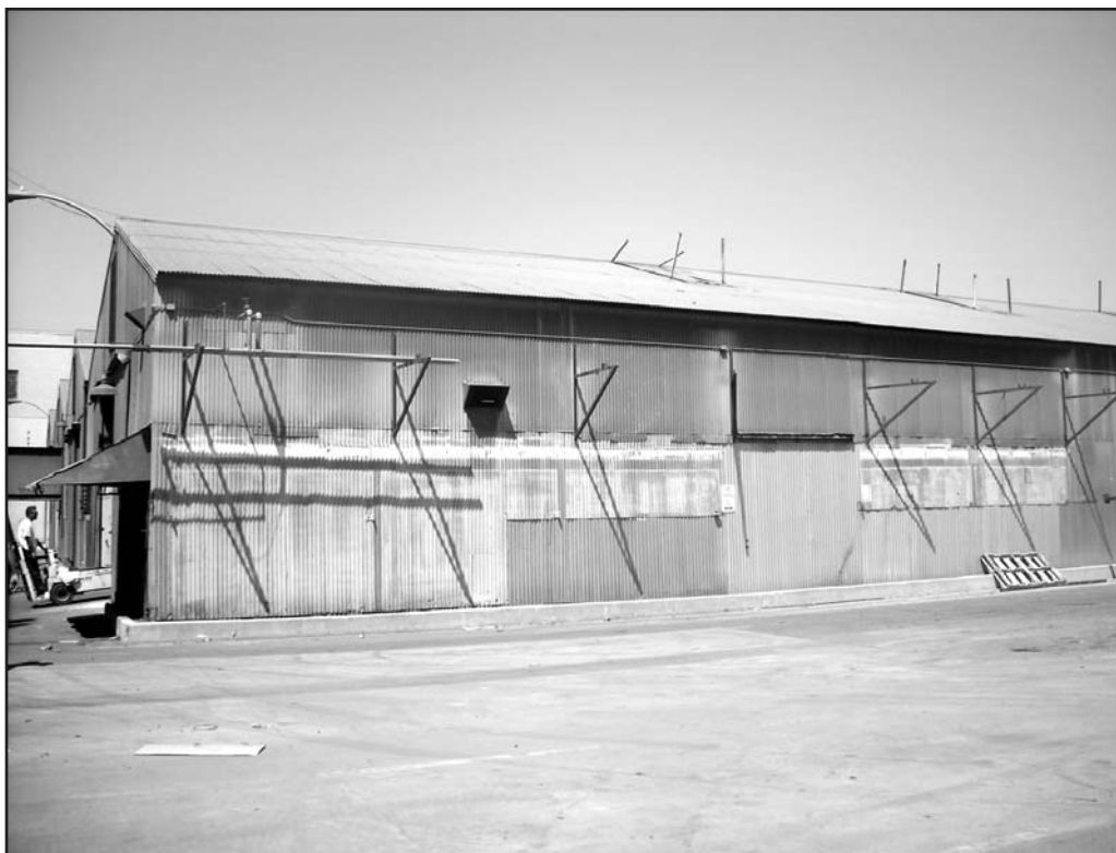
View of the north-facing facade of Building 3 located on the western project site.
