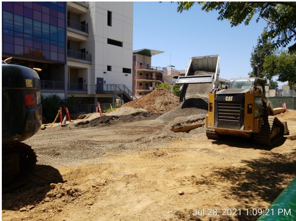
Retention Tank Installation
